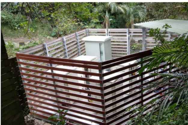
H<sub>2</sub> generator with 20 kW FC as UPS for mobile station.
