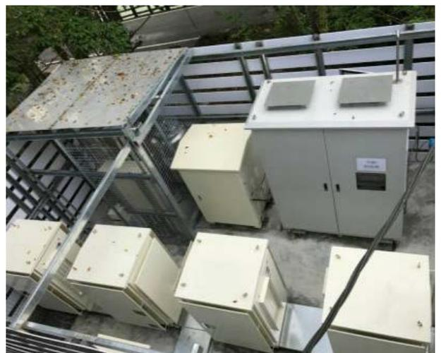
H<sub>2</sub> generator @20 NM<sup>3</sup>/hr with 20 kW FC to back up telecom facilities.
